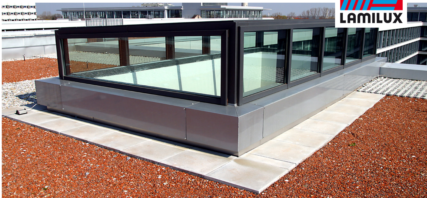
Parking facility, Schwabing
