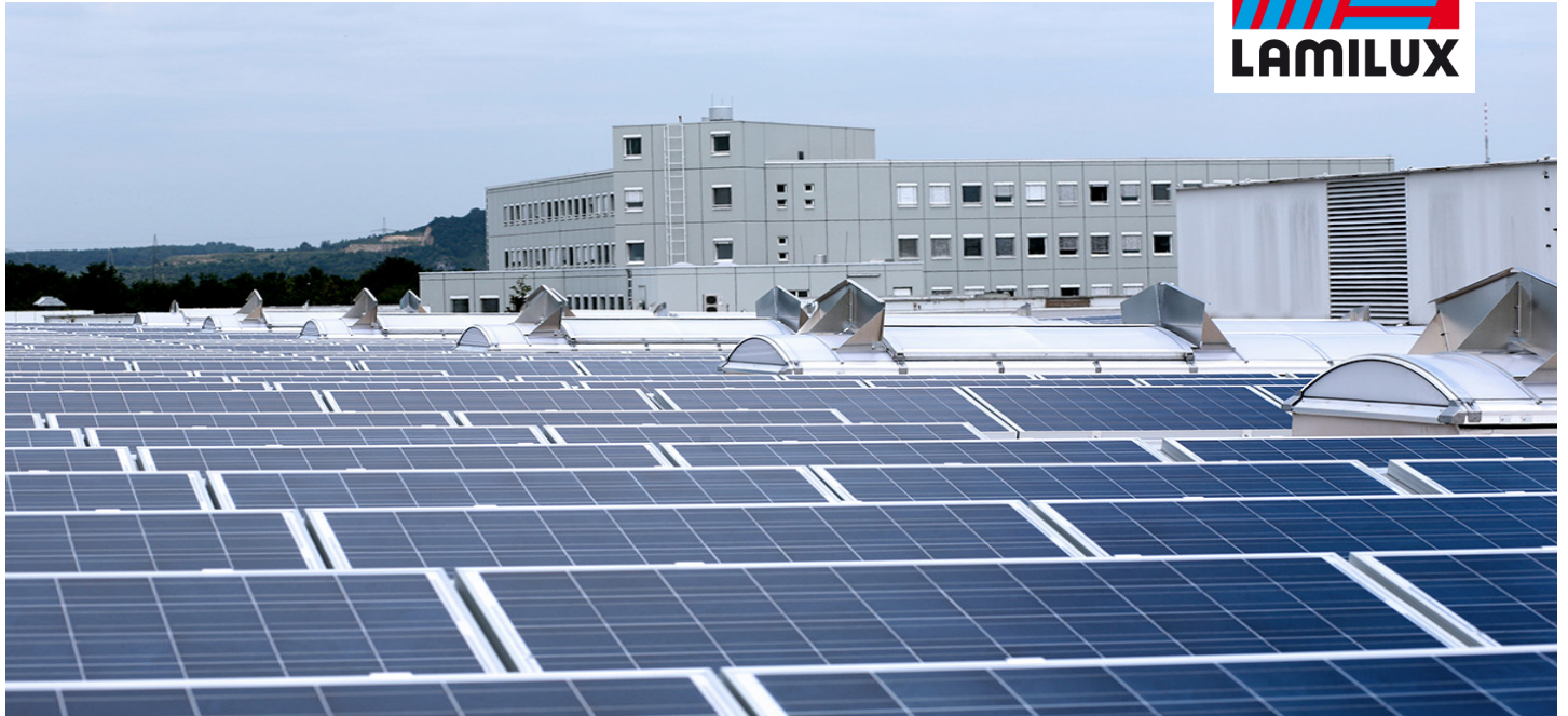
Schneider Electric, Regensburg, Germany
